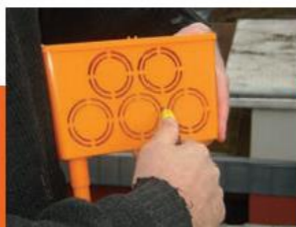
3/ Ouvrir le(s) opercule(s)
